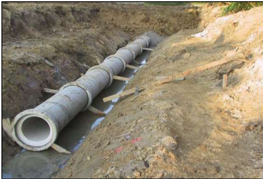
Fig. V.02. Conducts of concrete no armed.
