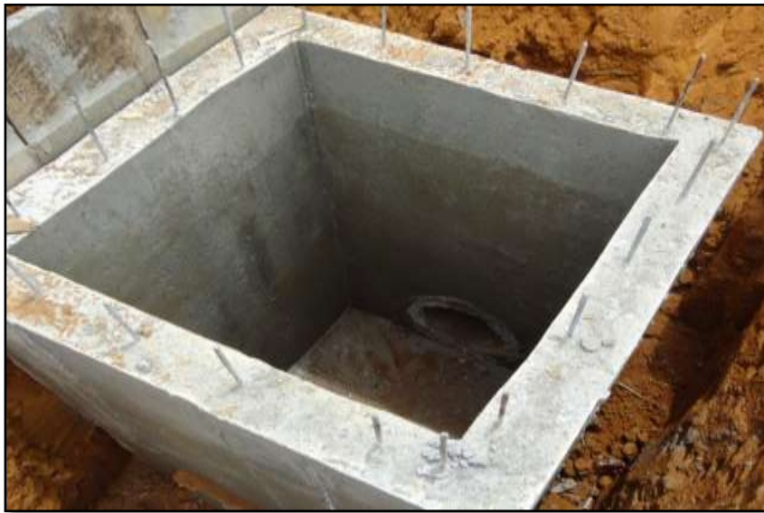
Fig. VI.01. Inspection manhole diagram.
