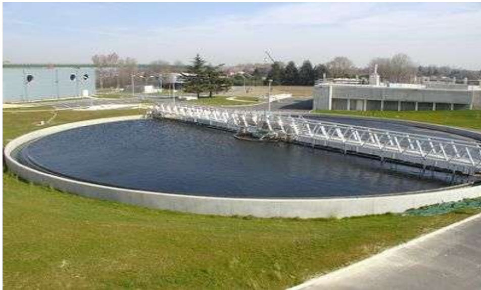
Fig. VI.10. Example of a settling basin. [ 10 ]
