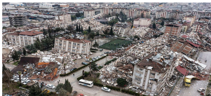
Figure 1.1: An aerial view of collapsed buildings in the Turkish city of Hatay [5]
