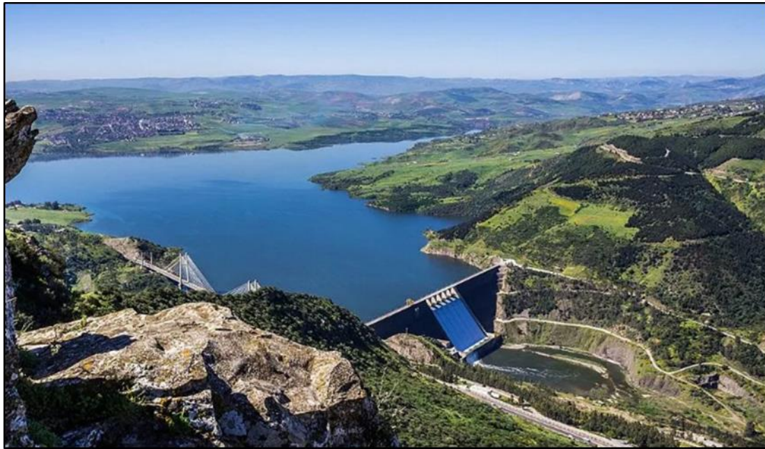
Figure 9 : Barrage de Beni Haroune 2020 (Site)
