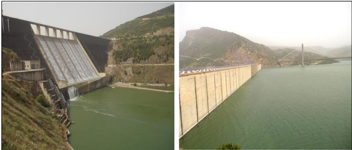
Figure 27: Beni Haroun Dam within the state of Mila (Remini, june 2014).
