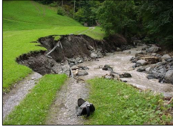
Figure I.4 Erosion des berges.
