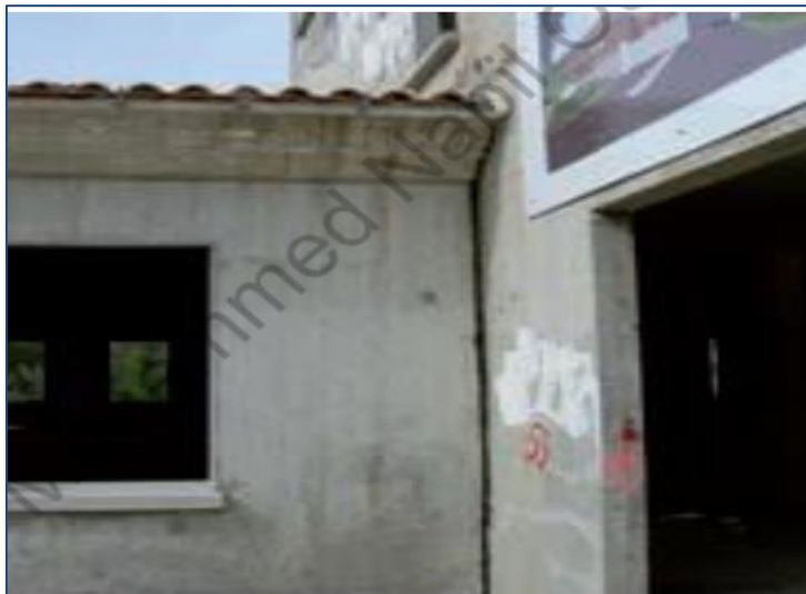
Figure II.11: joint sismique
