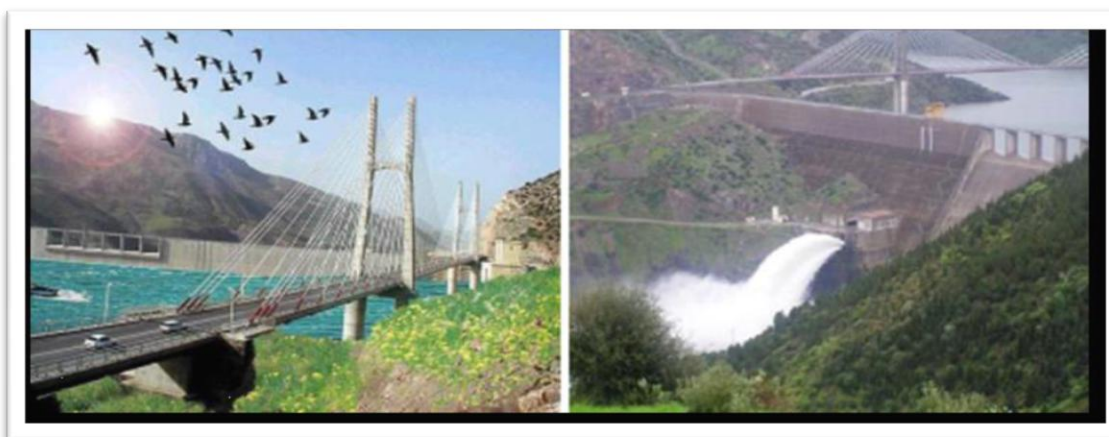
Fig. 24: The Beni Haroun dam (Abid, 2014).
