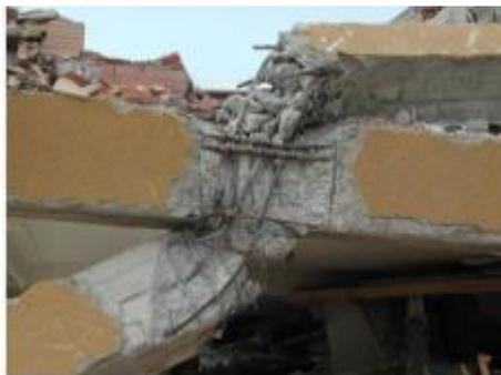
Figure II.12: Rupture en zone nodale. [4]
