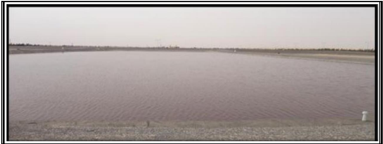
Figure III.9: Lagune de finition
