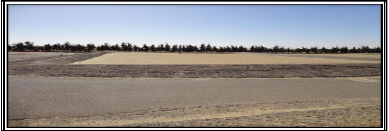
Figure III.10: Lits de séchage
